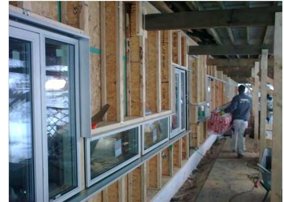
*Above: Old insulation has been removed and new windows have been installed
