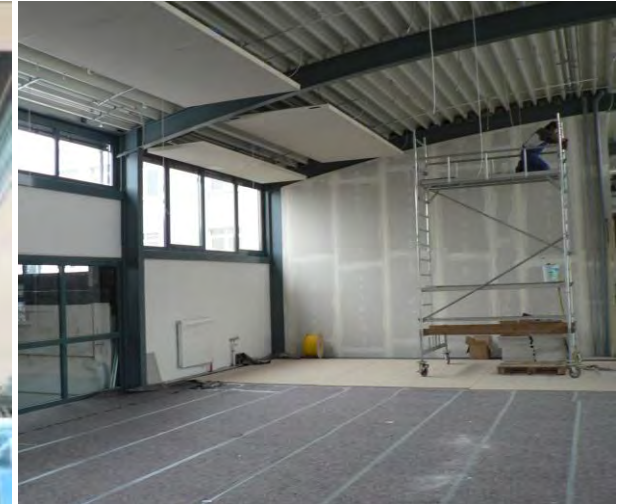
radiant-cooling sytem with phase change material
