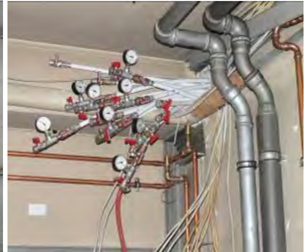
pressure test of the hydraulic system
