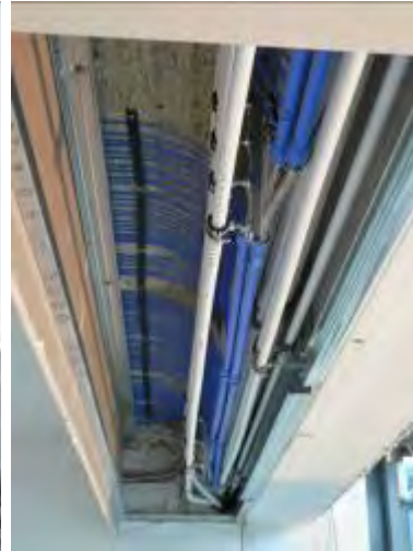
capillary-tube cooling system
