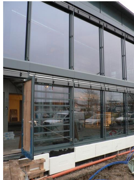
Façade with ventilation slats and solar shading system.
