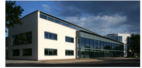
After retrofitting: building enlarged by a second floor: 1,110 m 2 , new building envelope is a light-weight steel construction
