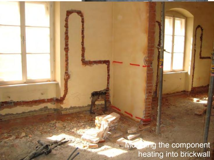
Mounting the component heating into brickwall
