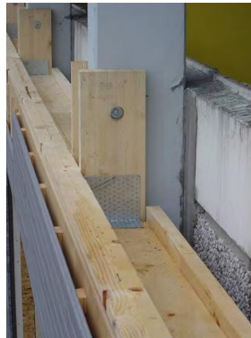
Mounting of façade elements
