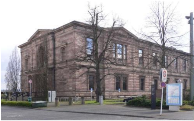
View from North West before renovation
