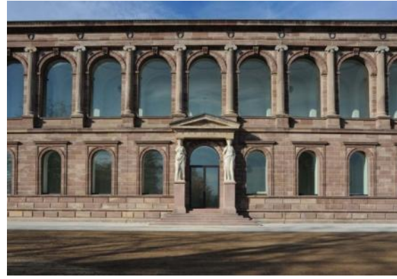
East façade after renovation
