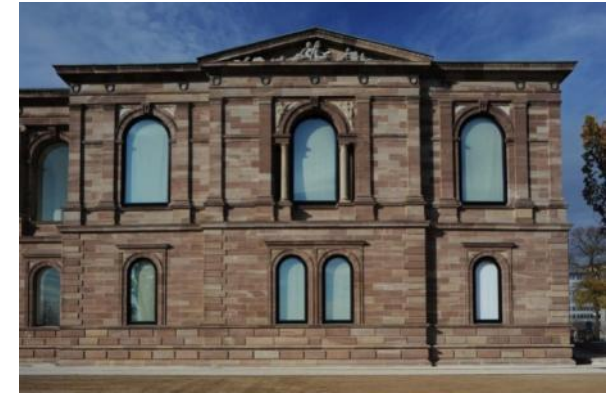
South façade after renovation
