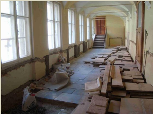
Foam glass insulation in the hallways. Source: AEE Intec
