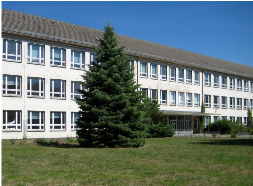
View before retrofitting
