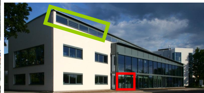
building after retrofit
