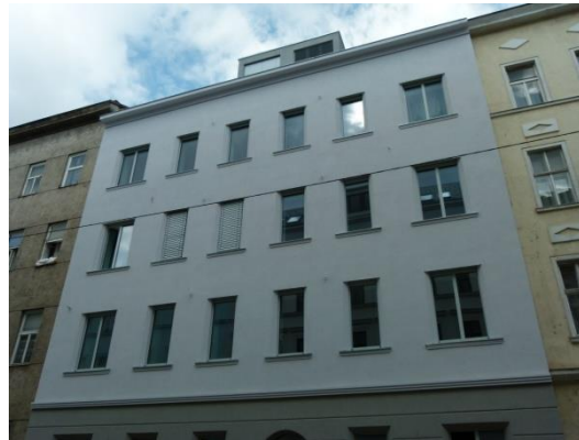
Object Eberlgasse, 1020 Vienna - First modernization of a historic building to passive house standard - water/water heat pump - air ventilation system
